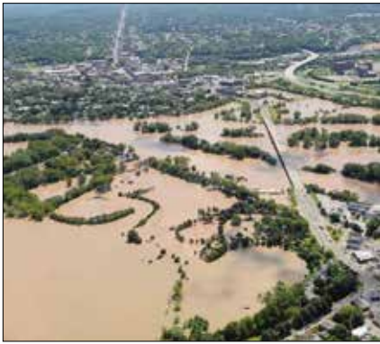
This aerial photo depicts the impact of Tropical Storm Irene in the Schenectady, N.Y., area in 2011.
